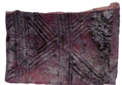
Box-flue tile with scoring to help adherence of plaster
